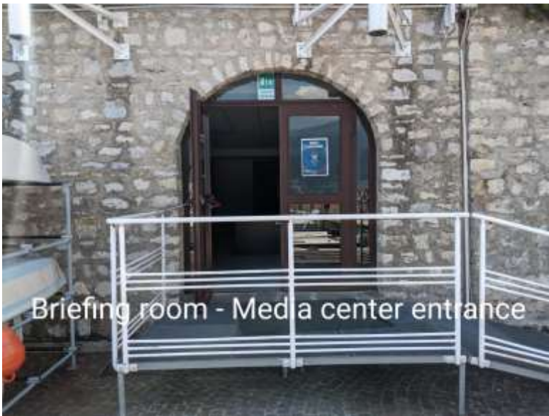
Briefing room Media center entrance
